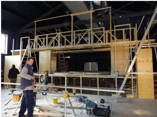
two meters and virtually the width of our theatre. The stage, which is totally demountable, has a large revolve and the facility for a front and back bridge 1.7m above the stage.
